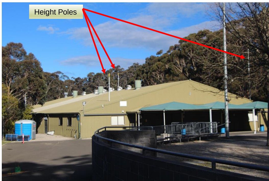
Figure 13 View of auditorium with height poles
