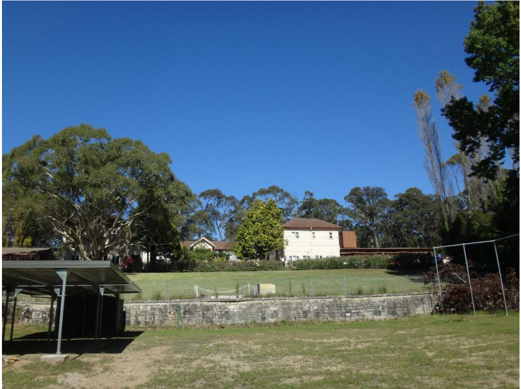
Figure 5 View of Clairvaux Accommodation building
